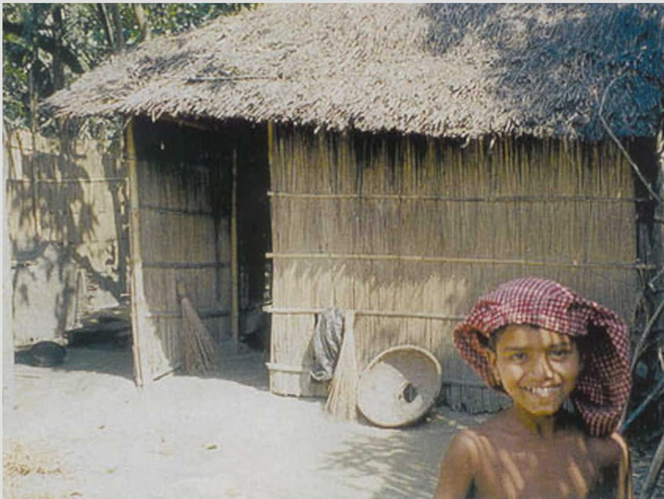
Traditional Bangladeshi jute hut, using local bamboo and a thatched roof.
